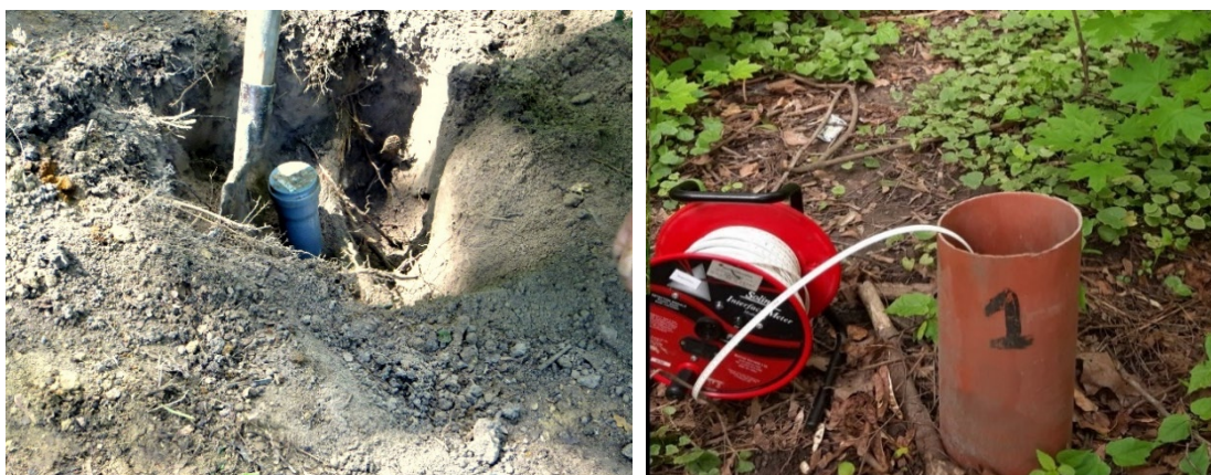
Fig. 3. Drilling of observation wells and measuring of water and petroleum product levels (2021)
